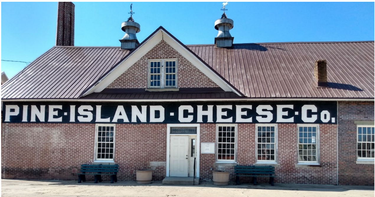
The Cheese Factory building near Trailhead Park.
